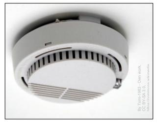
detectors are designed to effectively operate from fires involving "ordinary" combustible materials such as furniture, paper, and office décor while operating in clean building environments, special smoke detection systems are available for harsh environments and/or, for special hazards such as slow-growing electrical wiring fires typical of computer rooms.
